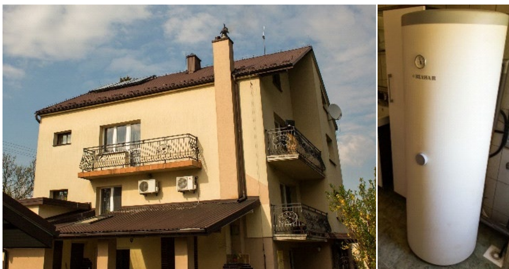
Fig. 1. The detached house and the solar storage tank inside Source: own study
