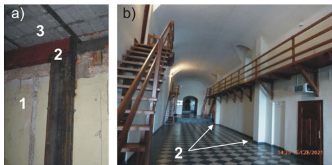
Fig. 9. Steel structures unloading the vaults in the east wing of the Dominican monastery founded on the transverse first floor wall: a) one of steel frames under construction, b) present view of the corridor in the second floor lined with the steel frame (1 – longitudinal wall standing on the vault, 2 – steel frame, 3 – ceiling above the second floor)
