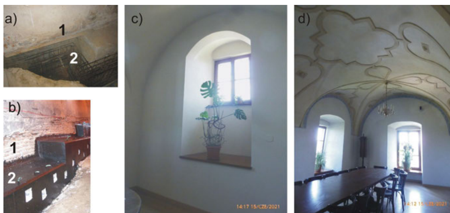
Fig. 8. South-east corner of the east wing in the Dominican monastery: a) and b) the micropiled structure supporting the corner – the internal and external grid beams photographed under construction (1 – east wall, 2 – micropiled structure), c) present view of the restored corner room in the ground floor (the wall shown in Fig. 3b), d) present view of the restored corner room in the first floor
