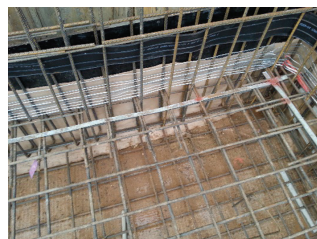
Fig. 6. System based on “rubber” joints (authors’ archive)
