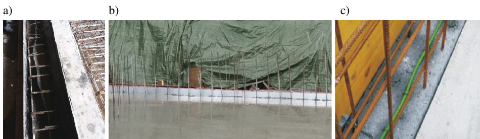
Fig. 3. Systems based on: a) “rubber” joints, b) “metal sheets”, c) injection hoses (authors’ archives)
