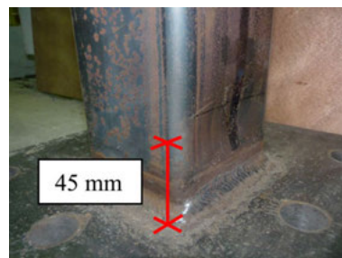
(d) Deformation of SHS-20 (right face)
