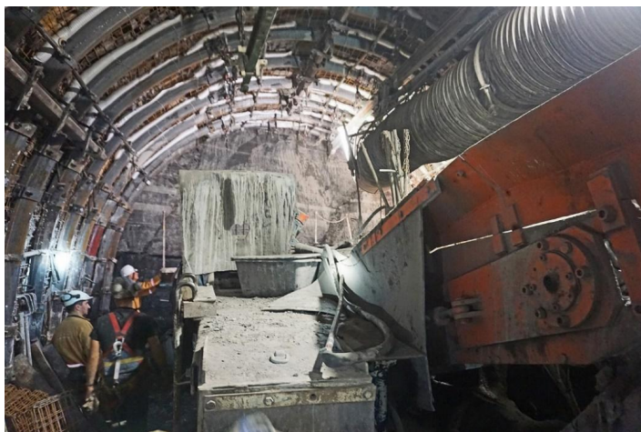
Fig. 1. View of the mining face of a gallery drilled with a roadheader
