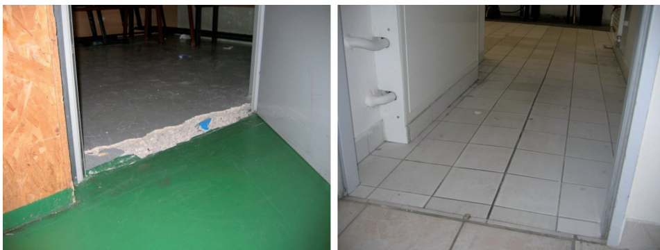
Fig. 4. Threshold failure caused by floor slab lift (left); Visible swelling of the floor with ceramic tiles (right)
