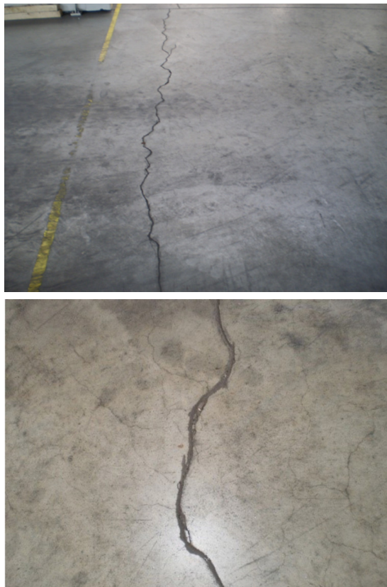
Fig. 2. Cracks of the industrial floor near the entrance to the production hall
