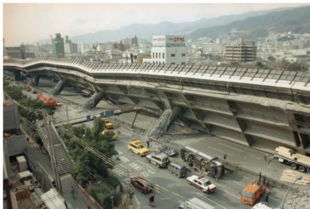
Fig. 1. Failure of a flyover on the “Hanshin” expressway after the 1995 Kobe earthquake source: https://www.japantimes.co.jp/opinion/2020/01/16/editorials/learned-enough-1995-kobe-quake/
