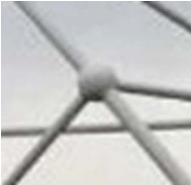
Fig. 4. Photograph of a typical node ball in a structure
