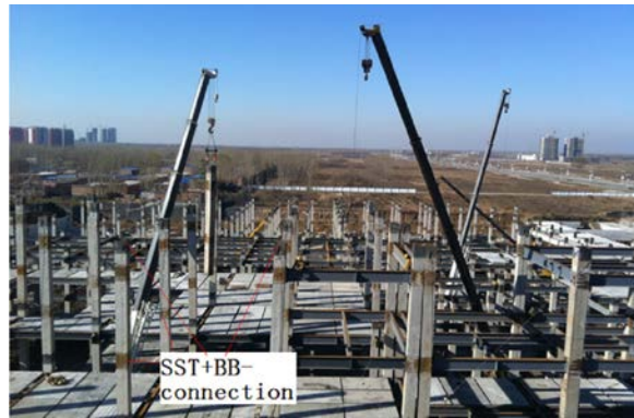
Fig. 1. SSPBB connection in practical project
