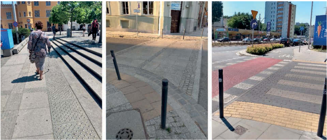
III. 4. Sample solutions that support the accessibility and safety of pedestrian routes in the centre of Wrocław: A) a pavement along the pedestrian access from the Main Railway Station to the public transport junction; B) a crossing on Włodkowica Street — extension of the pavement surface; C) a crossing on Prosta Street — raised crossing surface. Photo by A. Szewczenko.
