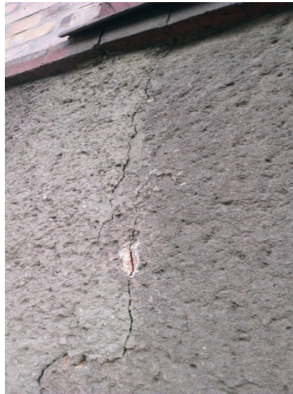
Fig. 12. Vertical cracking in the central part of the facade wall of Building A ( source: own work )
