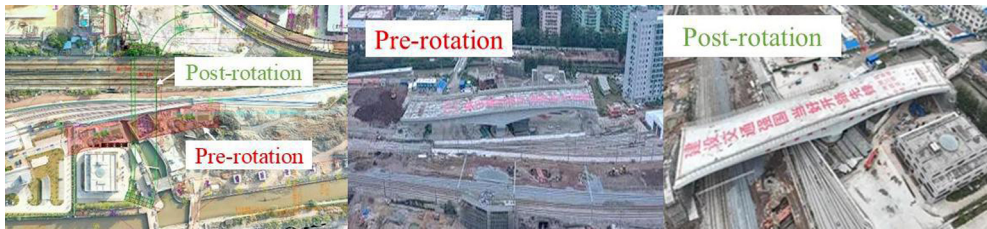
Fig. 9. Arrangement of the rotation construction
