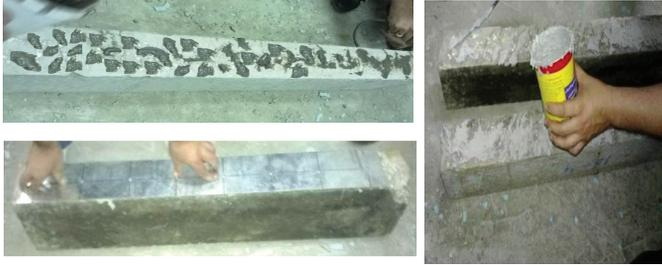
Fig. 7. Fixing the steel plate strengthening layer
