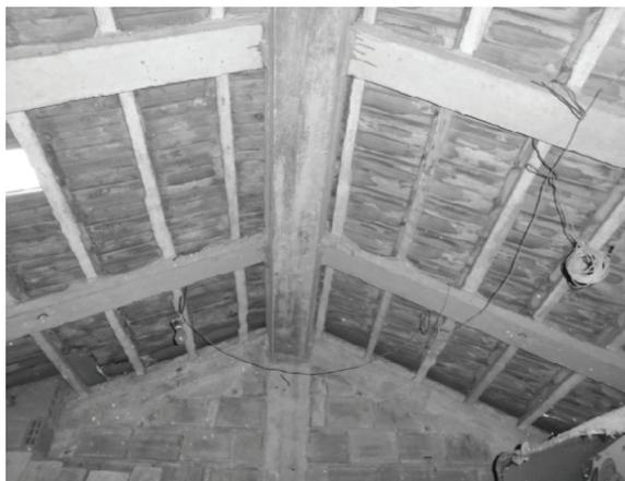
Fig. 17. Covering Structurally Supported by Prefabricated Beams
