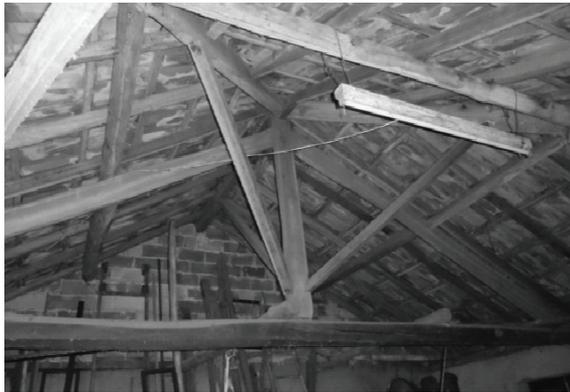
Fig. 16. Covering Structurally Supported by Wood Trusses
