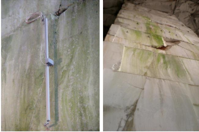
Fig. 9. Vertical EL beam gauge installation on the high safety pillar VS3 in Lipica II. quarry
