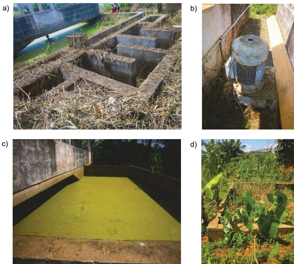
Photo 4. View of the abandoned treatment plant of CHU: a) pretreatment tank, b) turbine, c) aeration tank, d) sand bed; (phot. G.A. Ajeagah)
