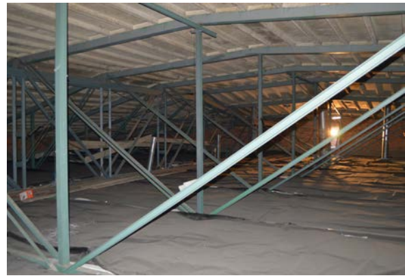
Fig. 10. Inside the ceiling of church VM.
