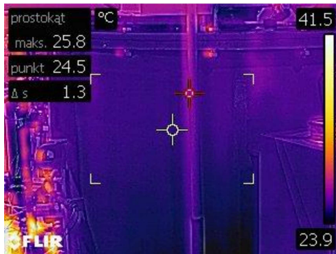
Fig. 3. Thermographic investigation of the shell of a vacuum furnace.
