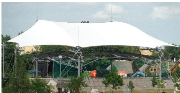
Fig. 1. Membrane hanging roof in Pruszcz Gdanski
