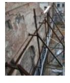
Fig. 10 Protection of walls with steel supporting structure, own archive, 12.10.2015
