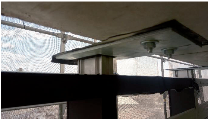
Fig. 1. View on fixed steel-aluminium brackets in mullion-transom wall system
