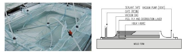
Fig. 1. VARTM process in Mostostal Warszawa [24] and the general scheme of VARTM production method [4]
