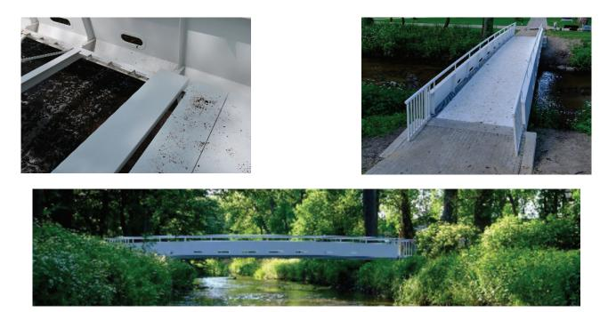
Fig. 16. FRP panels, top view and side view of the footbridge [8]
