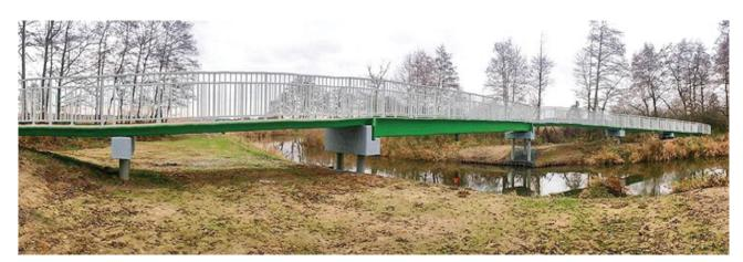
Fig. 11. Bicycle footbridge of the Dutch InfraCore system in the commune of Frombork [12]
