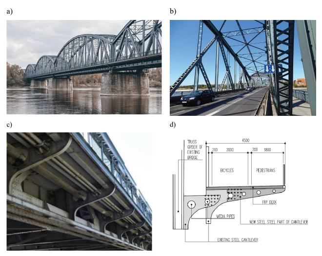
Fig. 20. The old cantilever and cross section of the new cantilever with FRP deck [15]
