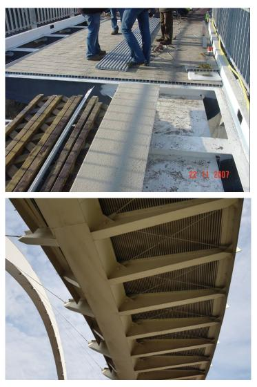
Fig. 15. Assembling of of FRP deck [6]
