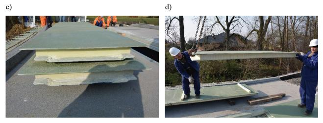
Fig. 17. Footbridge under construction and cross section of the main span with FRP deck
