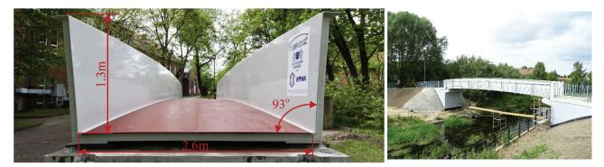
Fig. 7. Footbridge in Pruszcz Gdański: a) cross-section of the span; b) general view on site [1, 2]
