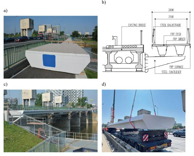
Fig. 19. Footbridge under construction and cross section of the cantilever with FRP deck
