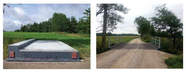
Fig. 8. Bicycle bridge of the Dutch InfraCore system in the commune of Lelkowo: half of the slab structure; finished object [12]
