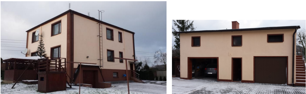
Fig. 10. Buildings # 1 and # 2 located in the zone of the convex curvature of the terrain ( Source: own study )
