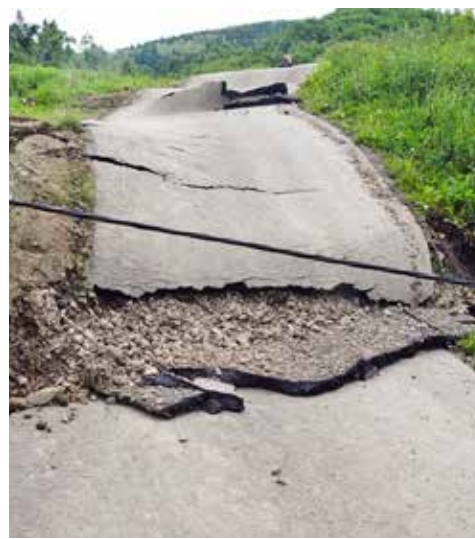
Devastation caused by a landslide in Kłodne, Limanowa municipality
