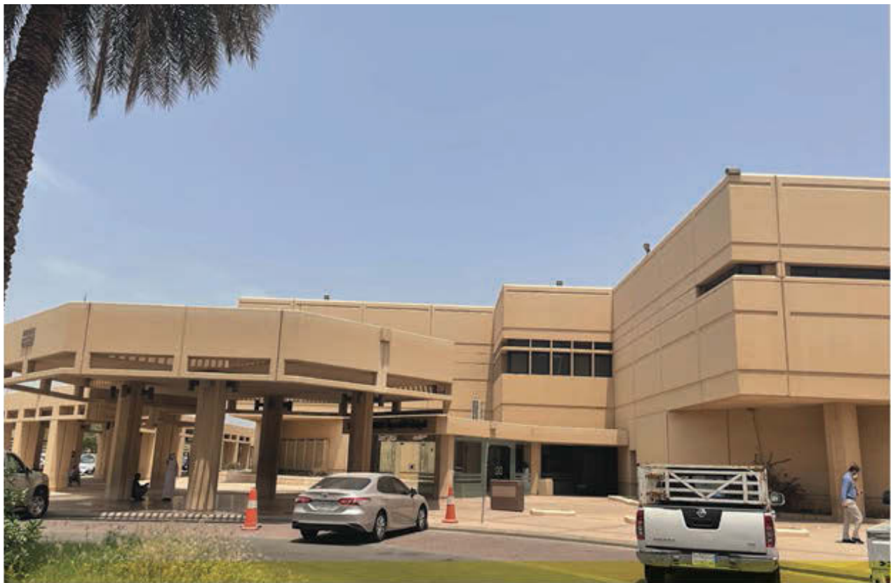
Ill. 4. King Abdulaziz University Hospital (KAUH), OPD building. Source: original work.
