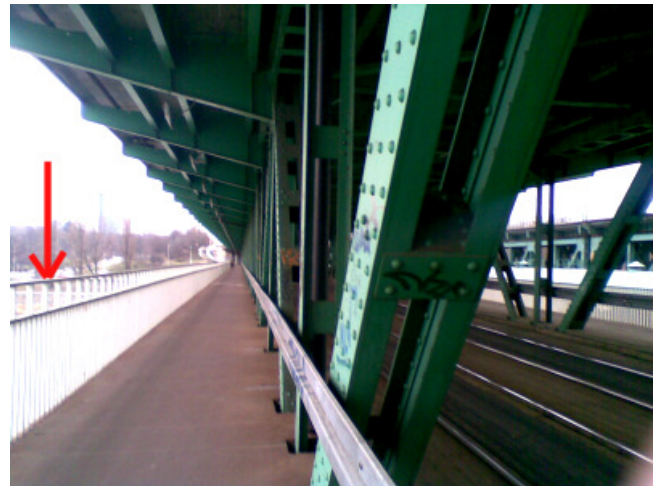
Fig. 7. Location of sensor on Gdanski Bridge in Warsaw.
