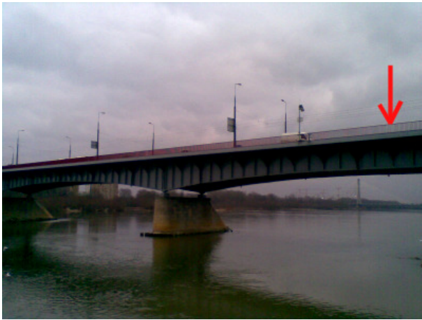
Fig. 10. Location of sensor on Lazienkowski Bridge in Warsaw.
