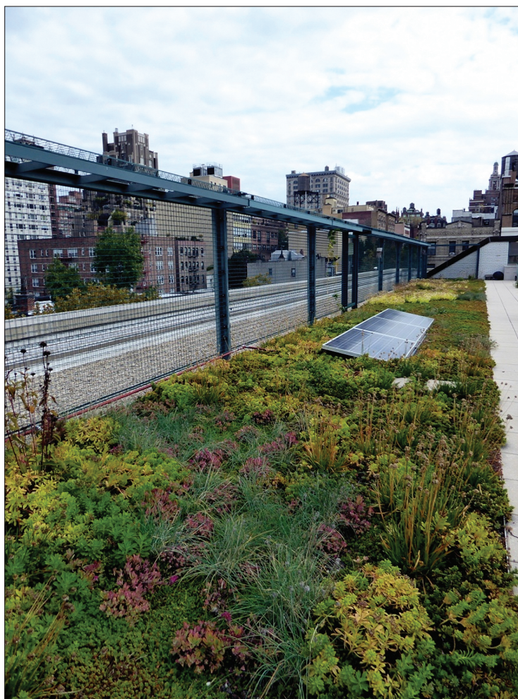
3. Zielony dach na Greenwich Village School w USA. Fot. Aloha Jon, 2016 r. 3. Green Roof on Greenwich Village School in USA. Photo by Aloha Jon, 2016
