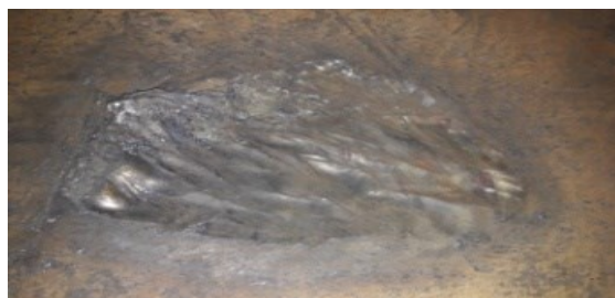
Fig. 1. Removing the defect by manual gouging
