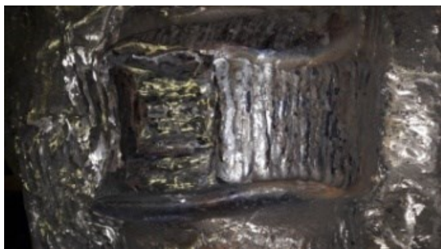
Fig. 7. Rebuilding of the surface of ladle by sequential welding
