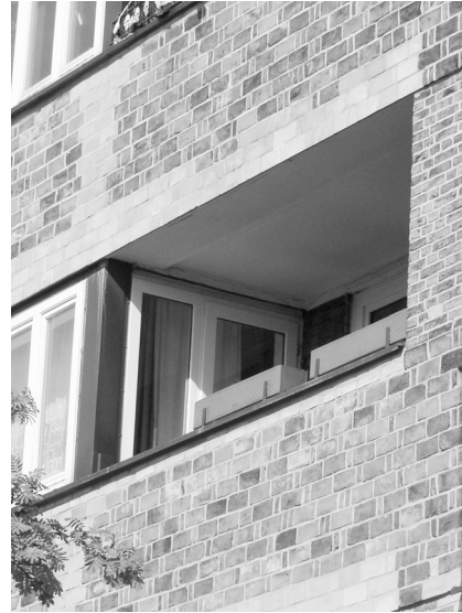
Photo 9. „Lunapark” multifamily complex – detail
