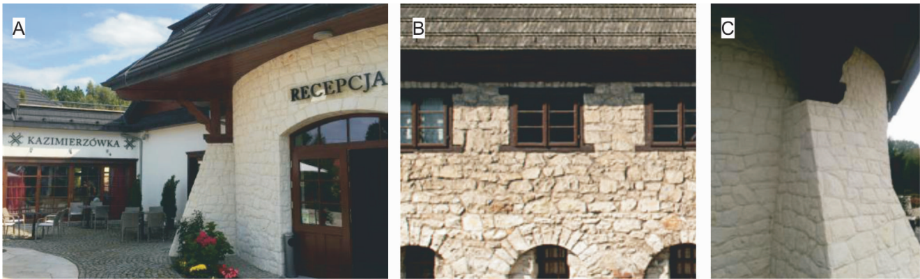
Fig. 7. A – Fragments of a modern hotel in Kazimierz Dolny; B – a renewed synagogue; C – a stylish retaining wall protected from rain and moisture.
