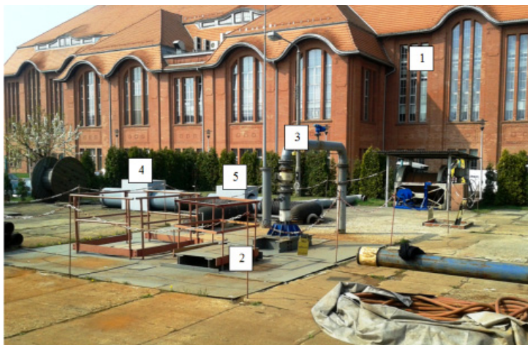
Fig. 2. The area of Gliwice II shaft. 1 – the building of Higher School of Economy in Gliwice, 2 – two symmetrical points of emission, 3 – pipelines for water pumps, 4 – the outlet of the fan no. 1, 5 – the outlet of the fan no. 2
