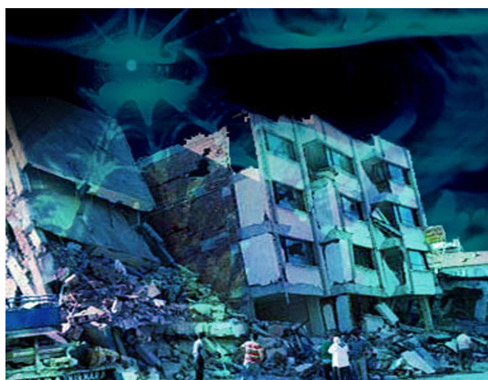
Fig. 10. Homes crumbled under the intense Kashmir Earthquake
