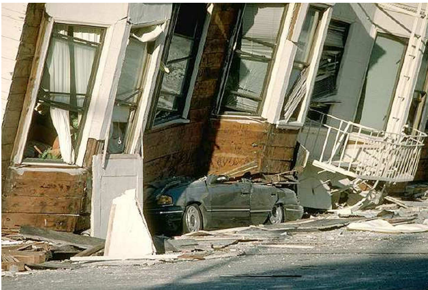
Fig. 5. A car is crushed by the collapsed row house
