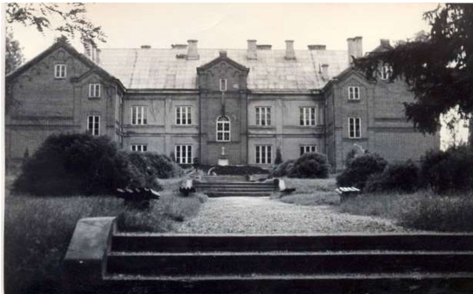
Fig. 5. The garden elevation of the Agriculture School in Sobieszyn and a part of the quartered garden, the 60s of the 20 th century [source: http 2 ]
