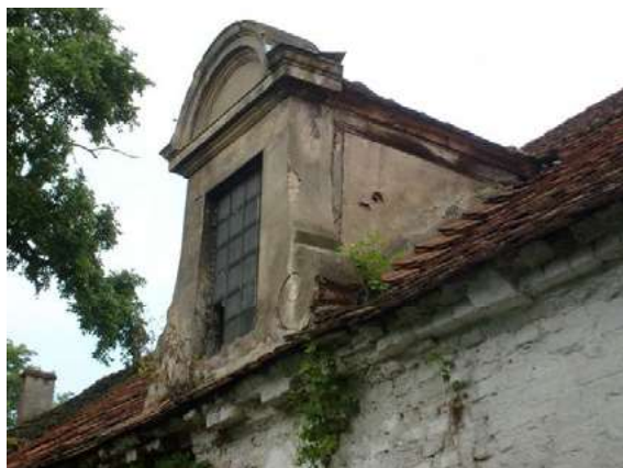
Ryc. 13. Lukarna na budynku, foto autorki Dormer on the building, photo author
