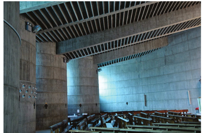
Fig. 3. Dispersive walls and roof structure.
