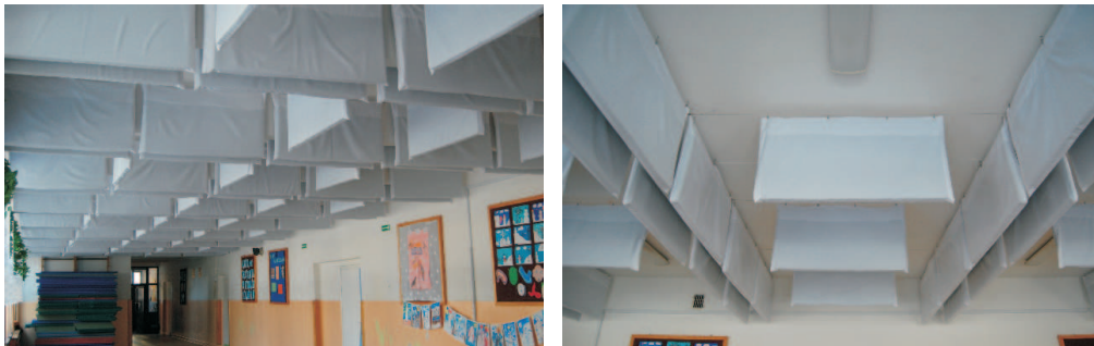
Fig. 1. School 1 corridor after acoustic adaptation.
