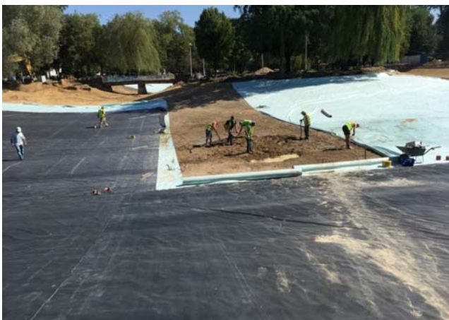
Photo 1. Profiling and sealing the bottom of the recreational reservoir (photo W. Walczak )
