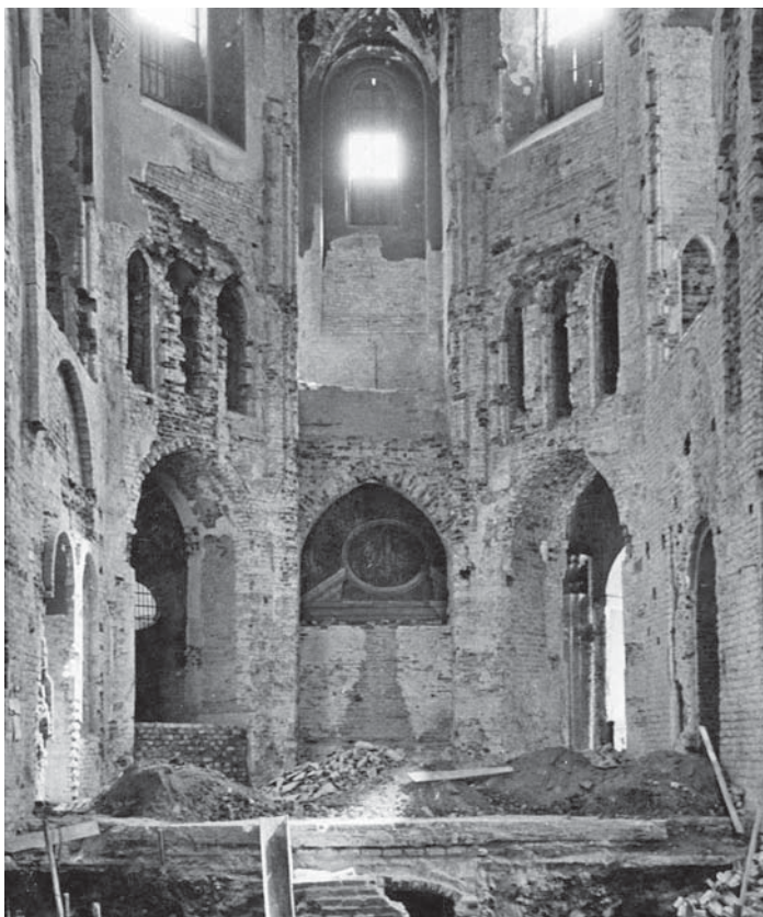
18. Poznań, cathedral, interior of the choir after the removal of the 18 th -century retablo of the main altar in 1948. Photo in the collection of the Municipal Conservator of Historical Monuments in Poznań
