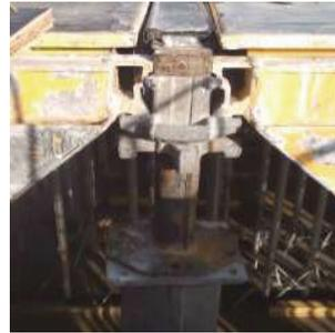
Fig. 4. CC-4 drop head in upper position [10]
