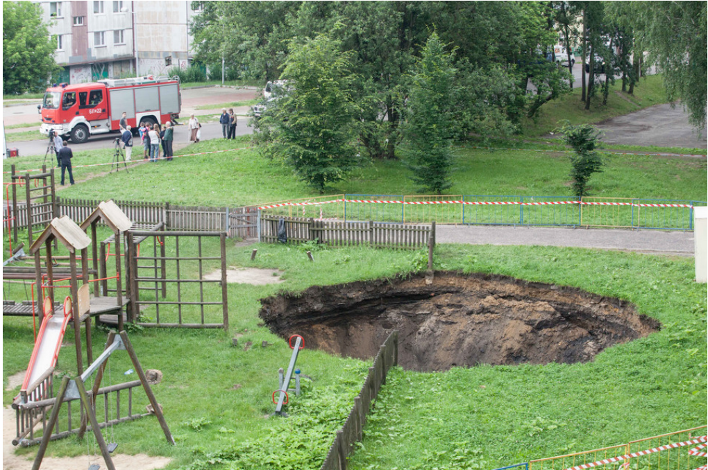
Fig. 2. Sinkhole in the former “Niwka Modrzejów” mining Area, Sosnowiec GZW Poland (Naszemiasto, 2013)
