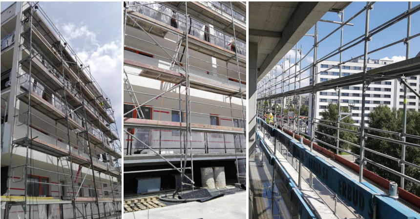
Fig. 1. Examples of the scaffoldings subjected to measurements
