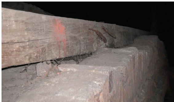
Fig. 11. Synagogue in Dąbrowa Tarnowska. Wooden truss bowstring loading the vault rib.
