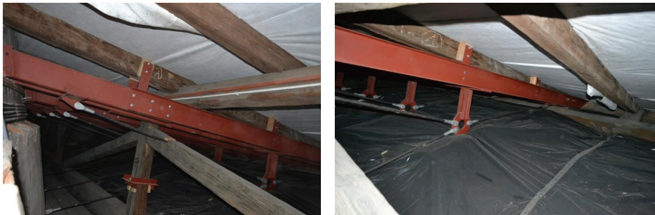
Fig. 8. Tension-strut system assembled in the attic of Lublin archcathedral treasury.
