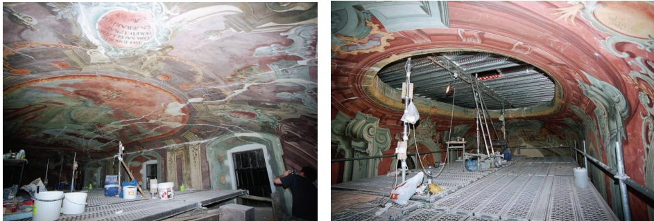
Fig. 7. Treasury of archcathedral in Lublin. Upper and lower vault during conservation.
