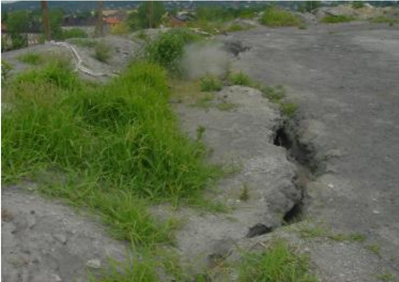
Fig. 8. Erosion crevice on a coal waste stockpile
