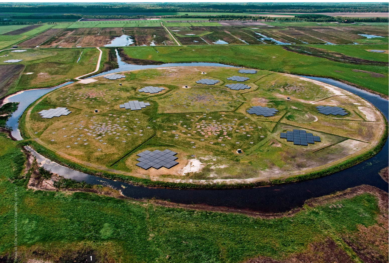
Fig. 1 The Superterp, the heart of the LOFAR core: six separate interferometer stations situated on an artificial island 320 m across. A further 18 stations are situated within a radius of 2 km, and another 14 within the whole of the Netherlands. There are a further 14 international stations (including three in Poland) and that number is continually increasing
