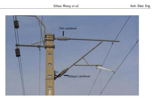
Fig. 1. Installation layout of cantilever insulator
