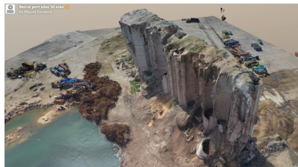
Fig. 7. The Beirut Port Silos 3D scan [36]
