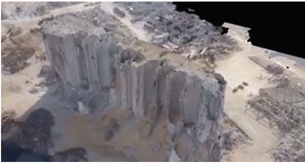
Fig. 8 The Beirut Port Silos 3D scan (open the link to access the video)
