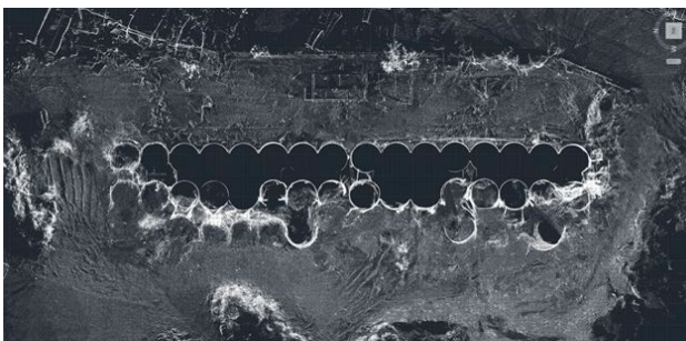
Fig. 6. The Beirut port silos- processed image from drone-mounted LIDAR scan
