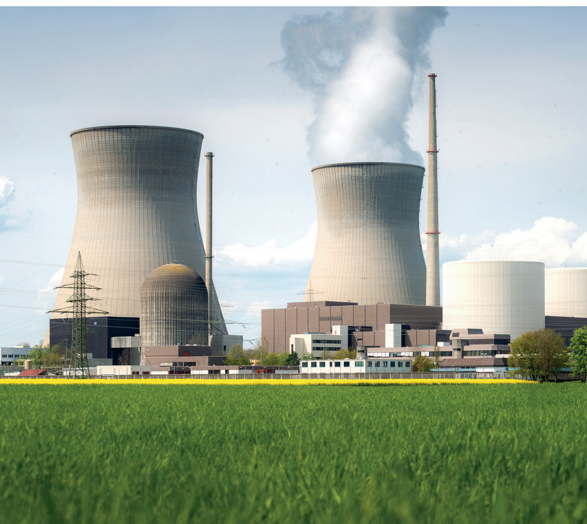
Nuclear power plant
