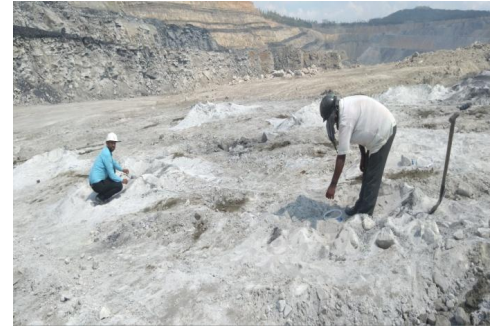
Fig. 4. Burden & spacing measurement
