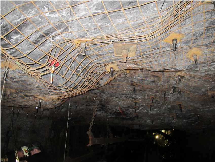
Fig. 11. The mine working (outby)
