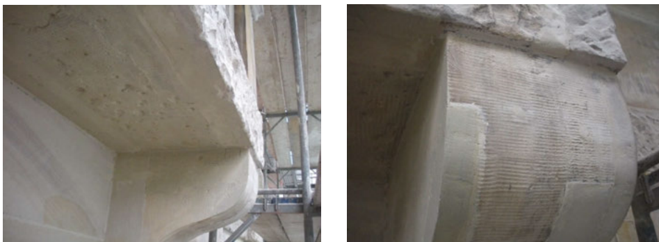
Fig. 13. Warsaw, Kredytowa street, 3. Strengthening elements covered with colour mortar
