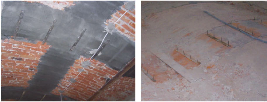
Fig. 5. School in Gorlice. Reinforcement of segmental barrel vault with FRP composite mesh. Bottom (left) and upper (right) sides of vault
