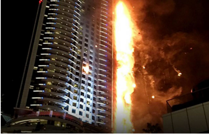
Fig. 2. Building's external wall cladding on fire in Address Downtown Dubai in 2015
